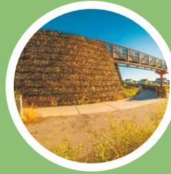
Gabions are used in transport construction on embankment slopes, as well as in the construction of artificial constructions - bridges and tunnels
